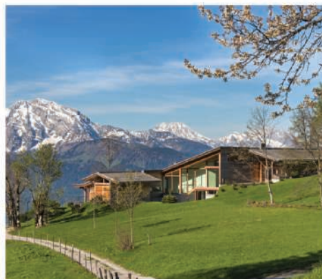
SALZBURG, AUSTRIA Exceptional villa with 360-degree views of the Saizburg Mountains and designed by the renowned architect Volker Hagen. Located 25 minutes away from the air-port, Featuring more than 600 sq m, this spacious country house is partitioned into a private living and sleeping area and an area for guests. Price upon request. Leo Hohla. Web: C55840 Stiller & Hohla +0043 662 6585 110
